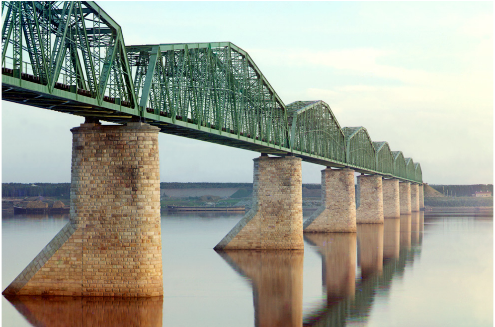
A metal truss bridge on stone piers, part of the Trans-Siberian Railway, crossing the Kama River near Perm, Ural Mountains Region, ca. 1910.
